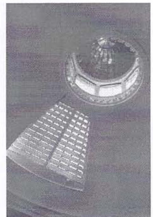
The louvered window in the Ether Dome helped illuminate the operative field in the days before electric lighting.
